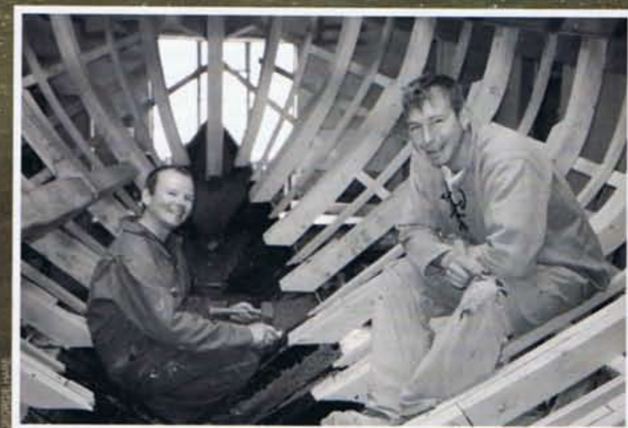
Ashley Butler (right) and Dave Showel put themselves in the frame during building
